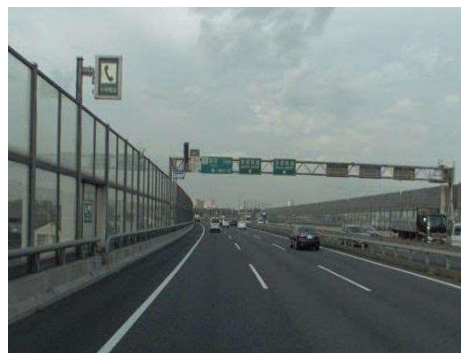
(Image during survey)
