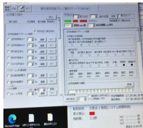
Traffic control center
