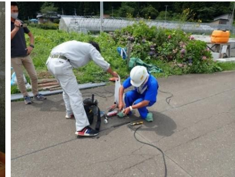
Recording infrastructure repair works to organize procedures
