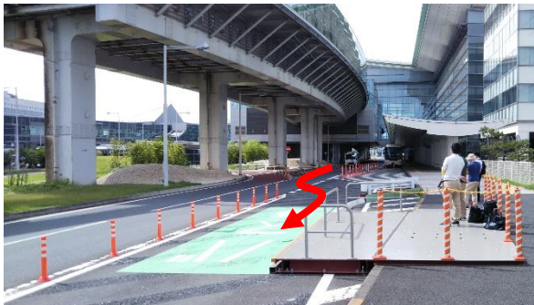
Terminal 3 bus stop
