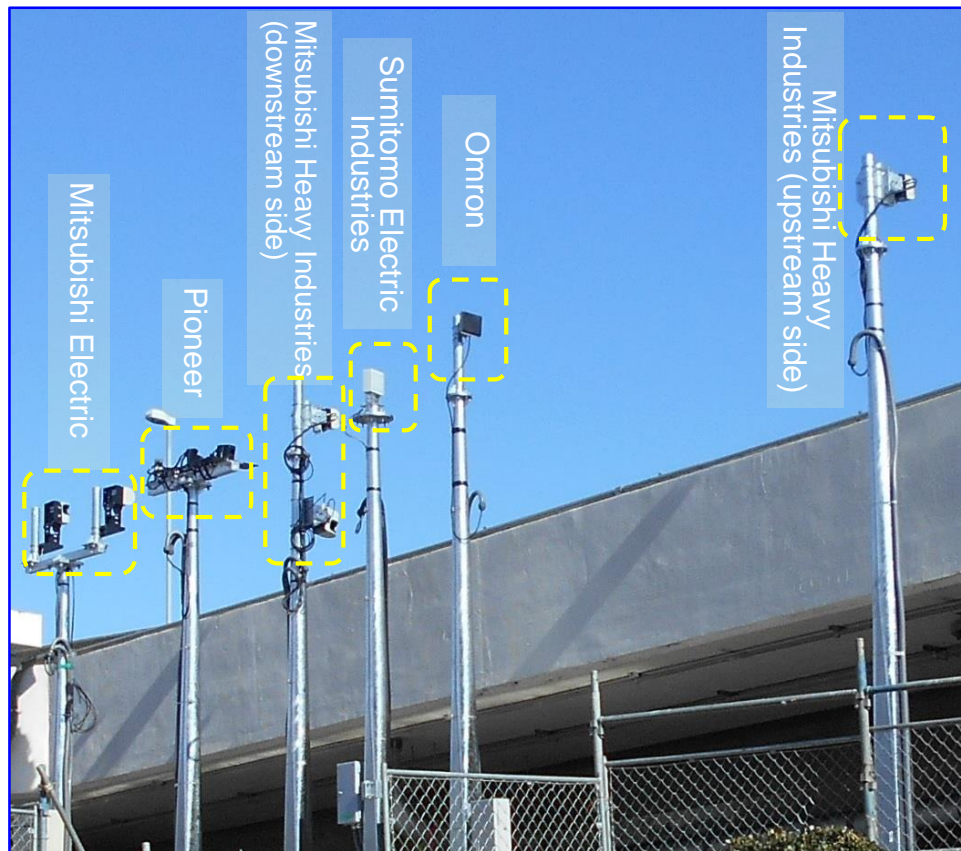
Figure 3-2 Sensor (1) installation (roadside sensors of five companies in NILIM joint research)
