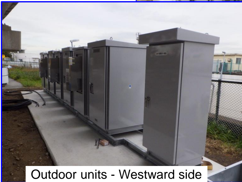
Figure 3-6 Appearance of outdoor units that house ETC gate passing support information provision management servers and processing roadside units of individual sensor manufacturers
