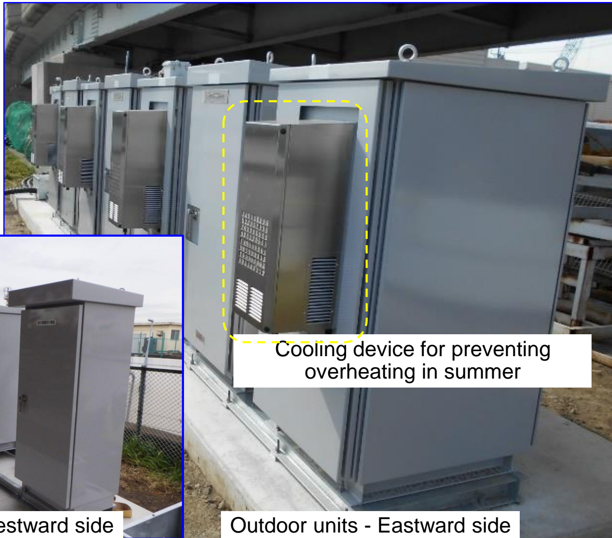
Figure 3-6 Appearance of outdoor units that house ETC gate passing support information provision management servers and processing roadside units of individual sensor manufacturers
