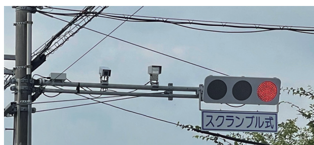
Fig.5 Various Sensors Installed on the Infrastructure Side
