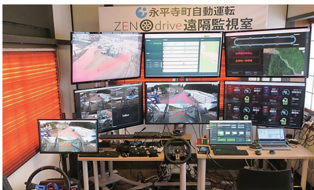
Fig.2 Remote Monitoring System in Eiheiji-cho
