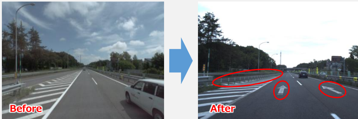
Example (2) Countersailing prevention measures at merging section (Addition of rubber poles and road markings)
