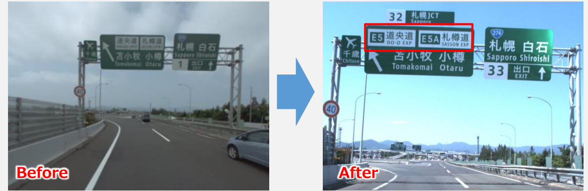
Example (3) Replacement of guide signs
